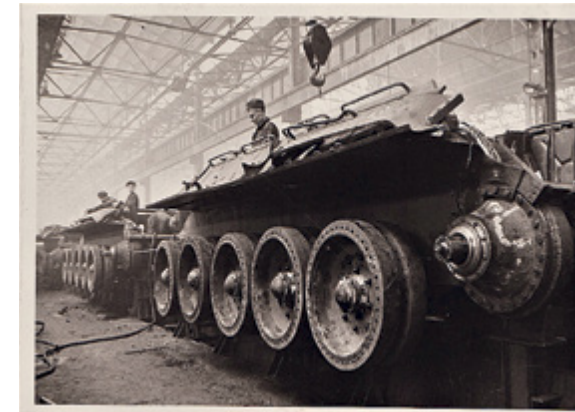
Assembly of heavy tanks
